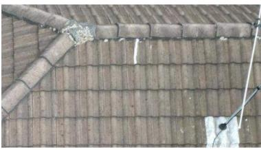
Gap in the hip capping tiles to be repaired/ sealed.
