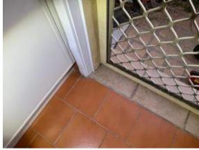
Rust to some steel door frames requires repair / repainting.
