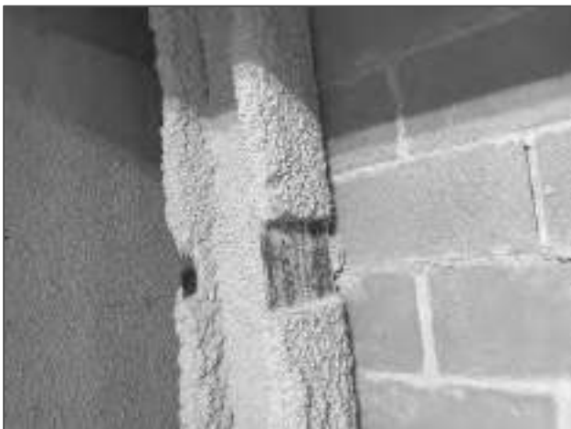
Photograph 3 –minor surface corrosion to the upper area
