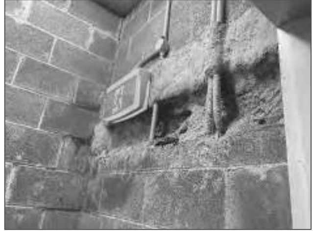
Photograph 13 – water marks and algae near the beam.
