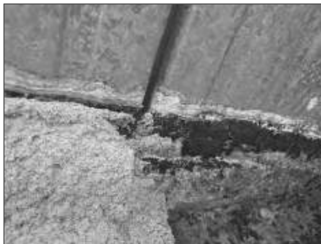
Photograph 27 – white oxide residue on the surface of the slab formwork-sheet system.
