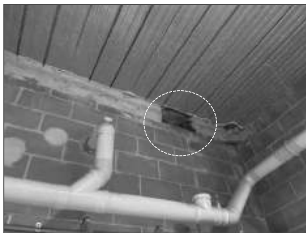
Photograph 25 – T6 after removal of the vermiculite coating
