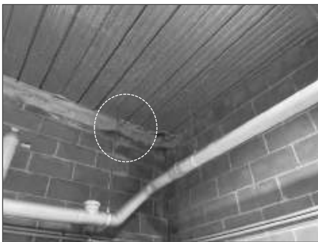
Photograph 24 – T6 before removal of the vermiculite coating
