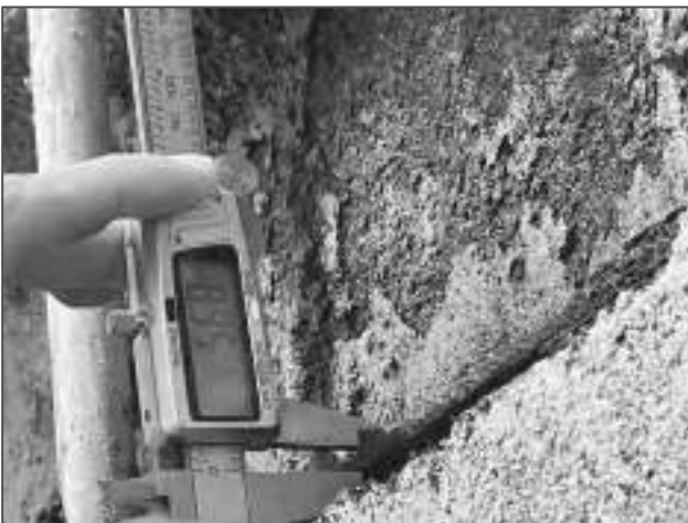
Photograph 16 – remaining thickness of the beam, 1 st reading
