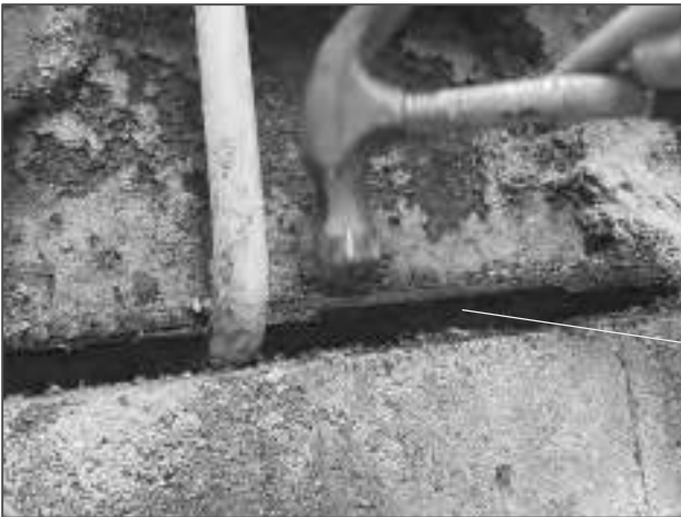
Photograph 14 – substantial material loss on the bottom flange
