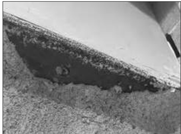
Photograph 21 – presence of surface corrosion on T5
