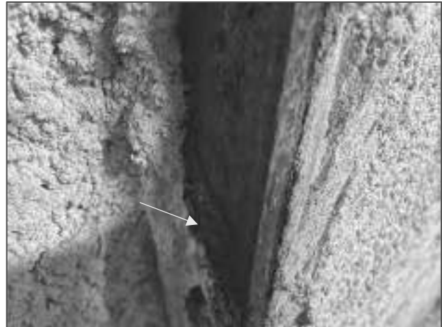
Photograph 2 – corrosion present at the base of the column
