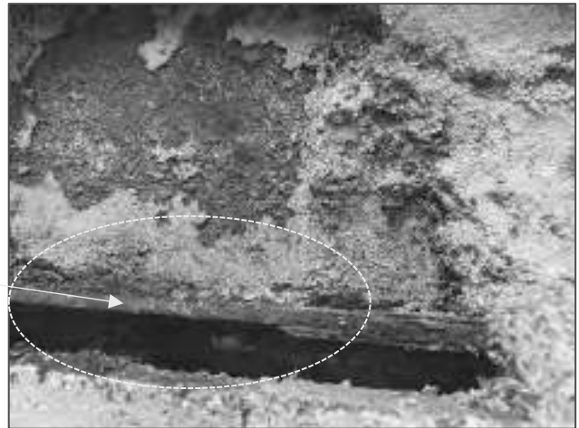
Photograph 15 – closeup image of the material loss on the bottom flange
