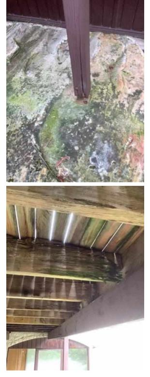
Some decking & framing timbers show signs of weather damage.
