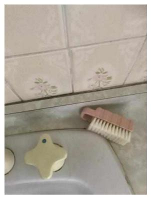
Junctions of bath and wall tiles require resealing with silicone.
