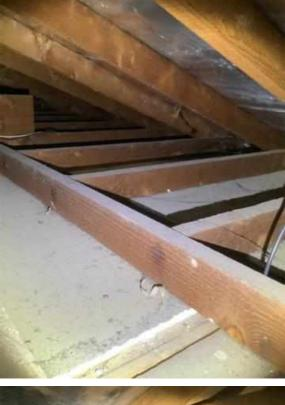
Evidence of termite damage to various framing timbers. Some of this damaged timber requires repair / replacement. We recommend a builder be engaged to determine a scope of work to rectify this damage. Refer to the attached Timber Pest Inspection Report.
