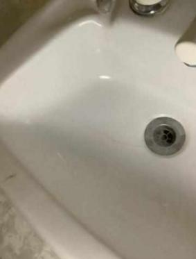
Cracking to hand basin requires repair/ replacement.
