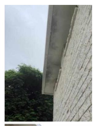
Some fascia / barge timbers show signs of weather damage and require repair / repainting.
