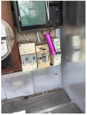
Note: Porcelain fuses have been identified to the switchboard. We recommend an electrician be engaged to remove the fuses and upgrade as required.
