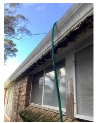
Some sections of gutter require cleaning.
