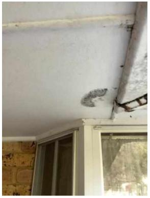
Some fascia / barge timbers show signs of weather damage and require repair / replacement.
