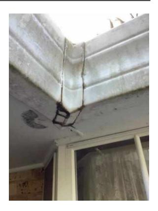
Some gutters are rusted and require repair / replacement.
