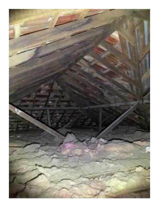
Signs of past water penetration was found in roof void I recommend a roof tiler or roofing plumber be engaged to find cause of leak and repair.
