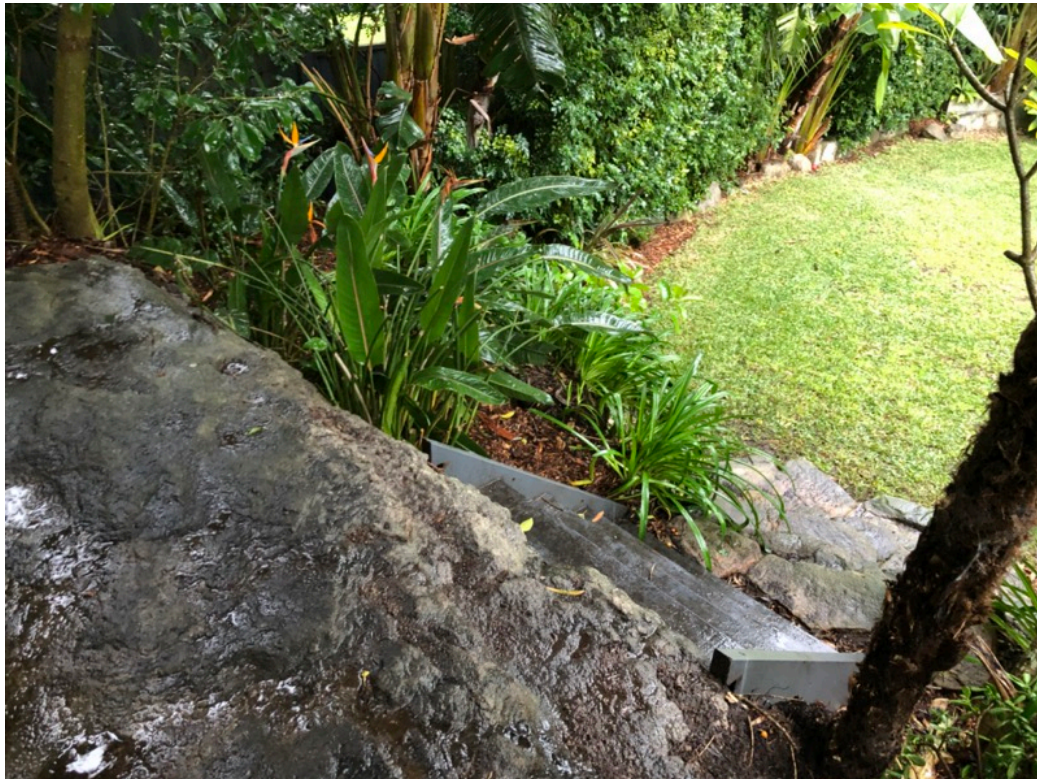
5. Fall hazard due to no handrail on backyard steps behind pool. Potential for injury.
