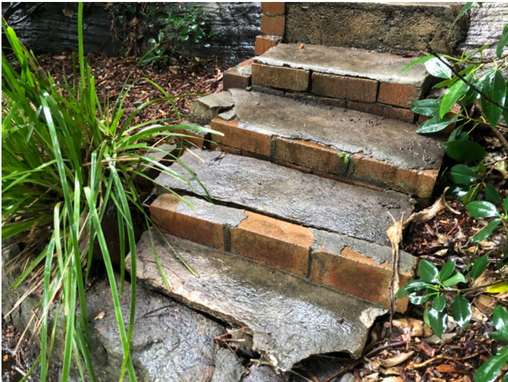
4. Loose concrete / brick step in backyard behind pool area. No further deterioration anticipated.
