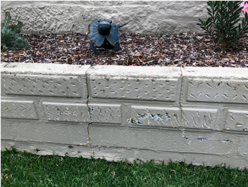
11. Garden bed crack near back yard steps. Appearance crack with potential for further cracking.
