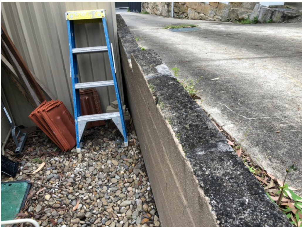
8. Leaning brick retaining wall on east side. Serviceability defect with potential for further deterioration.
