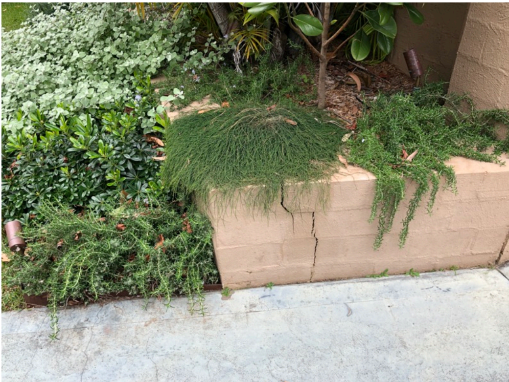
6. Garden bed crack near driveway. Serviceability crack with potential for further cracking.
