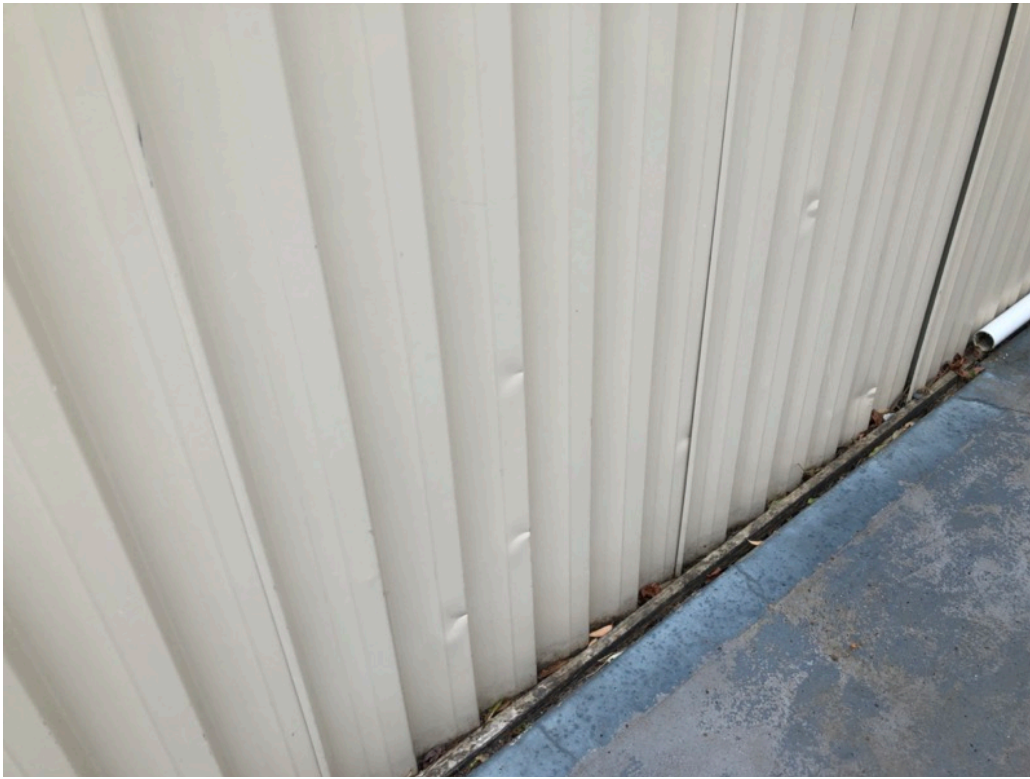
7. Multiple locations of dents to fence on west side. No further damage anticipated.
