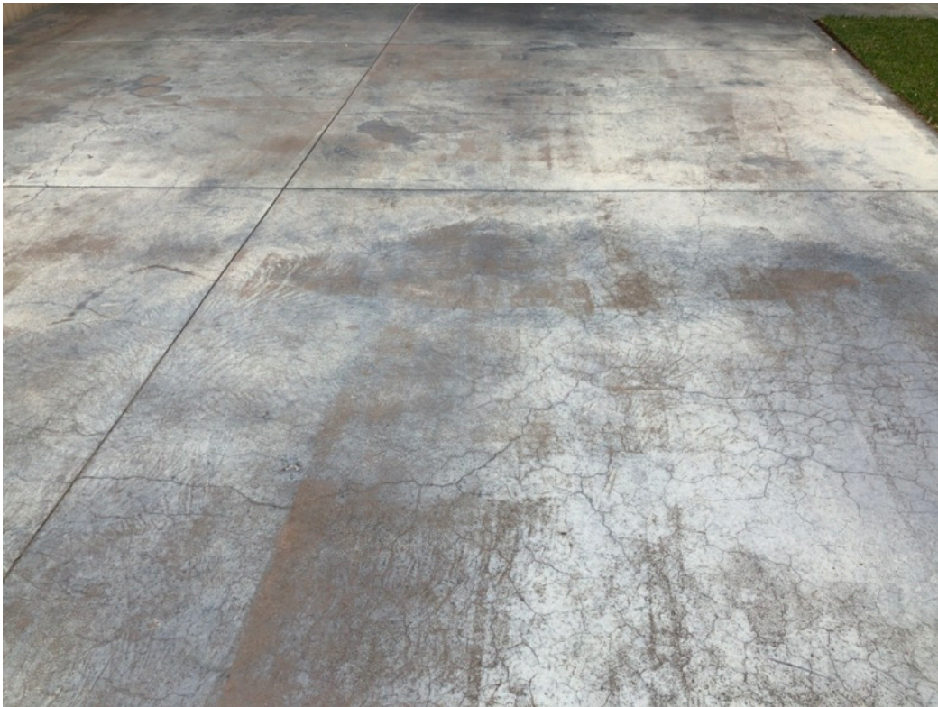
5. Webbed cracking to concrete driveway slab. Appearance cracks with potential for further cracking.
