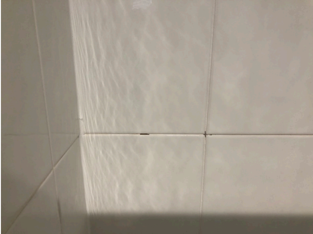
3. Grout deteriorating to wall tiles in shower of Ensuite. Potential for further deterioration.
