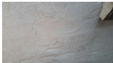
External cracks located to areas of this property.
