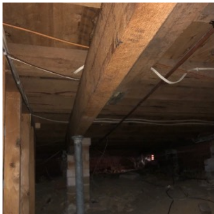
Brick piers with ant caps subfloor
