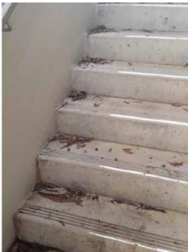
C 52 – Basement 1, south-east fire stair
