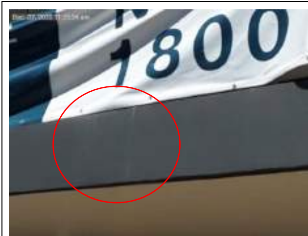
C 27 – East facade, balcony slab edge
