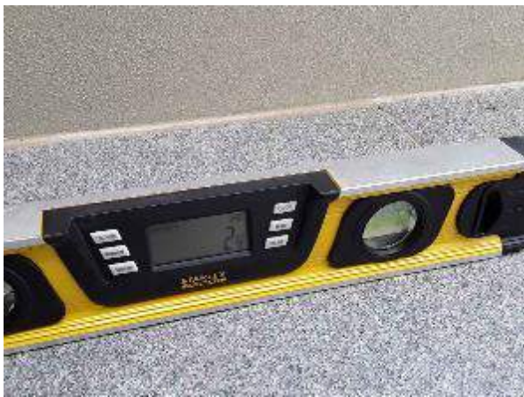
C 3 – G.floor north entry, floor tiles
