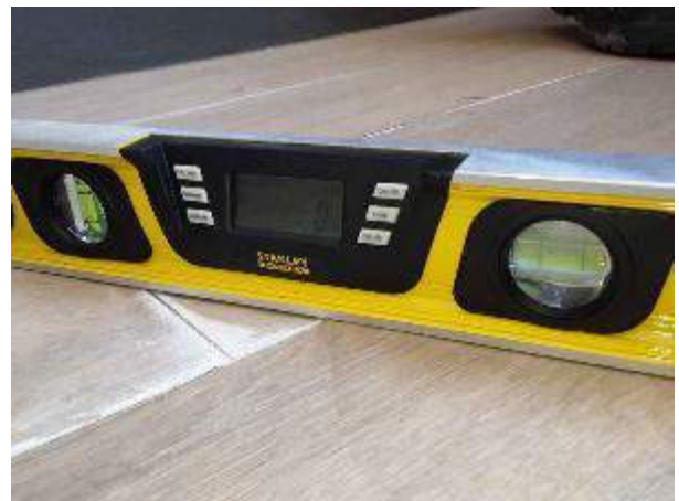
U 306.16 – Main bedroom balcony, floor tiles
