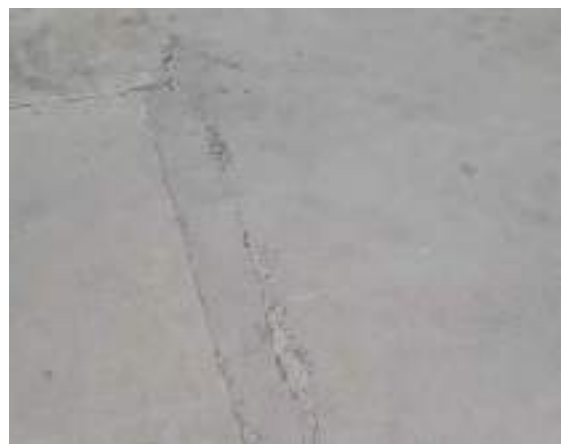
C 238 - Driveway, concrete slab
