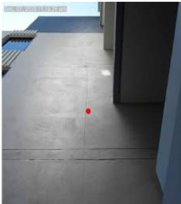
C 36 - West facade, Hebel cladding
