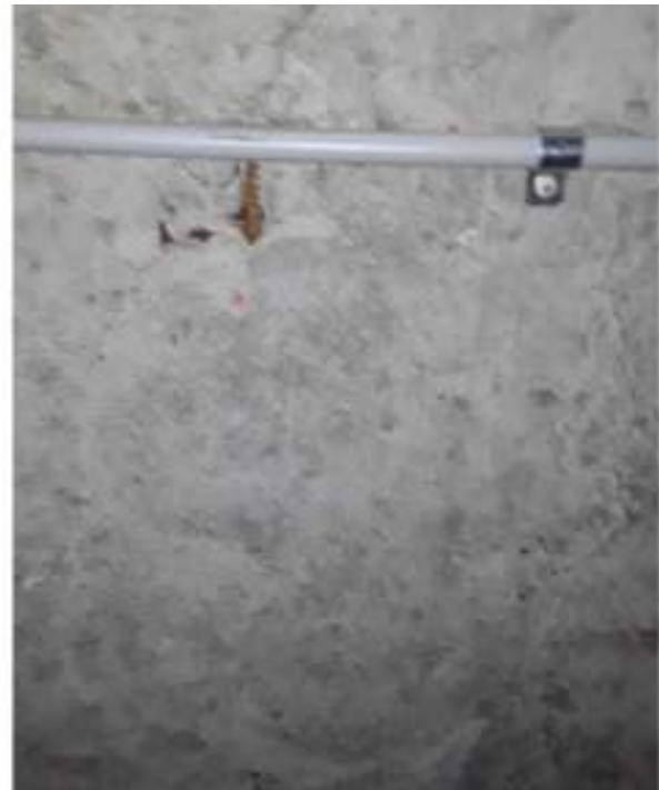
C 136 – Basement 2, north of building adjacent to ramp
