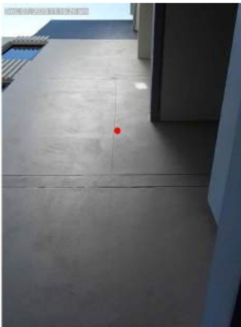
C 36 – West facade, Hebel cladding
