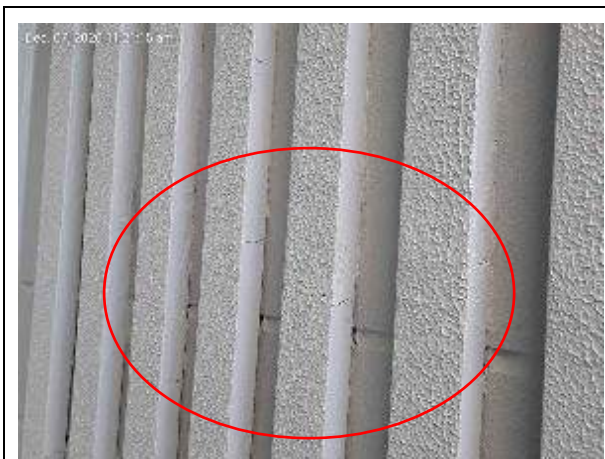
C 21 – East facade, Hebel cladding textured wall
