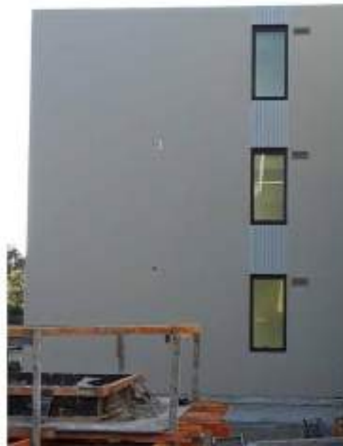
C 41 – North facade, Hebel cladding
