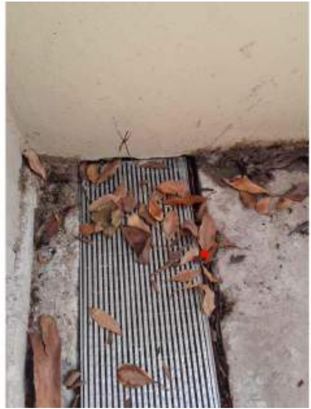
C 53 – Basement 1, south-east fire stairs to ground level
