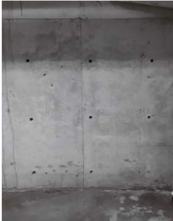
C111 – Basement 1, north-east fire stairs
