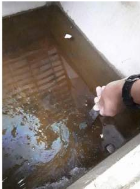
C 87– basement, hydrant room
