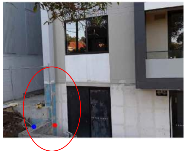
C 44 – South facade (Mitchell Avenue), Hebel cladding
