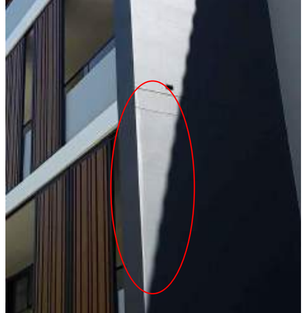
C 50 – South facade (Mitchell Avenue), cladding
