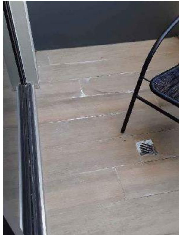
U 306.12 – Unit 306 Main bed balcony, floor tiles
