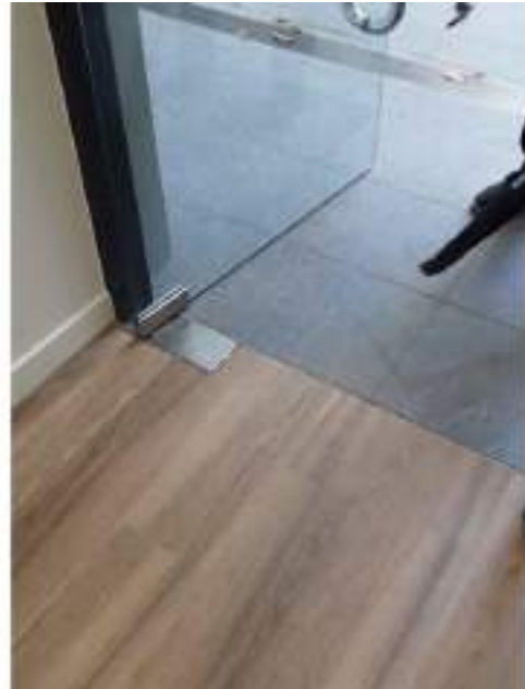
C 187 – Upper ground level, entry door threshold
