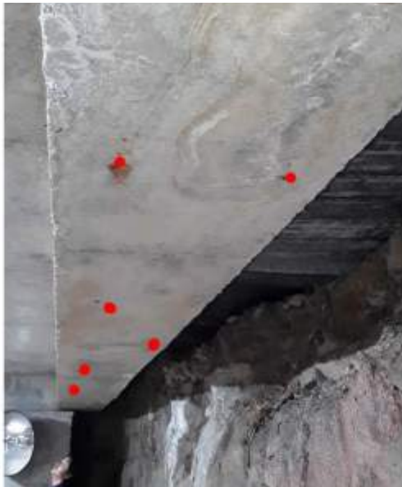
C 128 – Basement 2, north of building adjacent to the ramp
