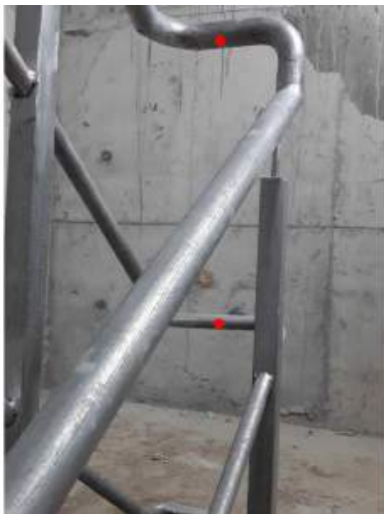
C 79 – Basement 1, north-east fire stair
