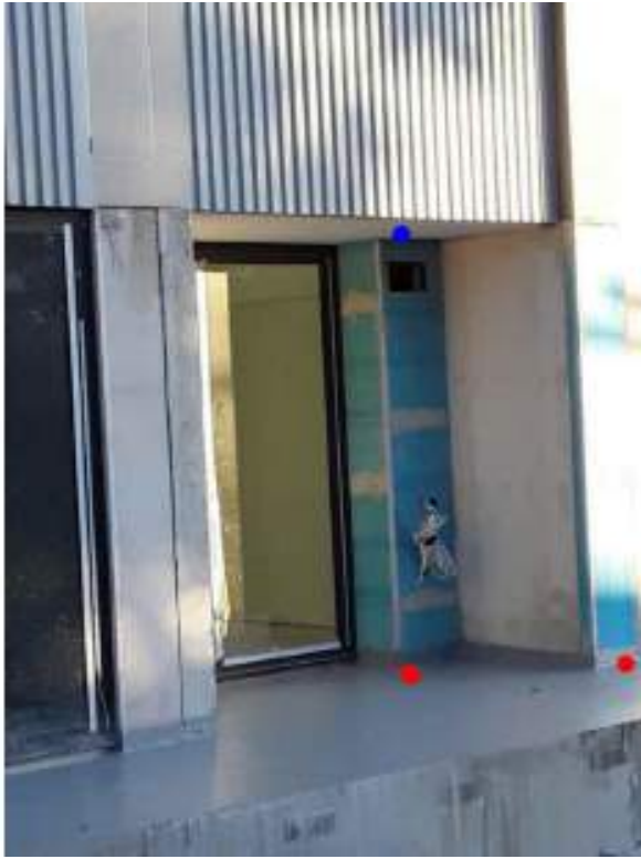
C 13 – East facade, unit balcony
