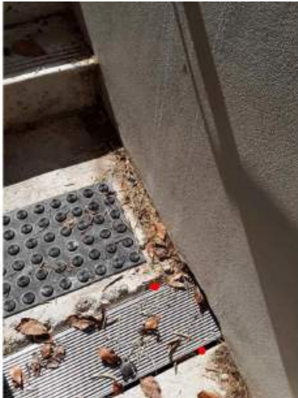
C 71 – Basement 1, north-east fire stairs to ground level
