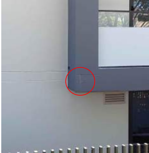
C 50 – South facade (Mitchell Avenue), balcony edge slab
