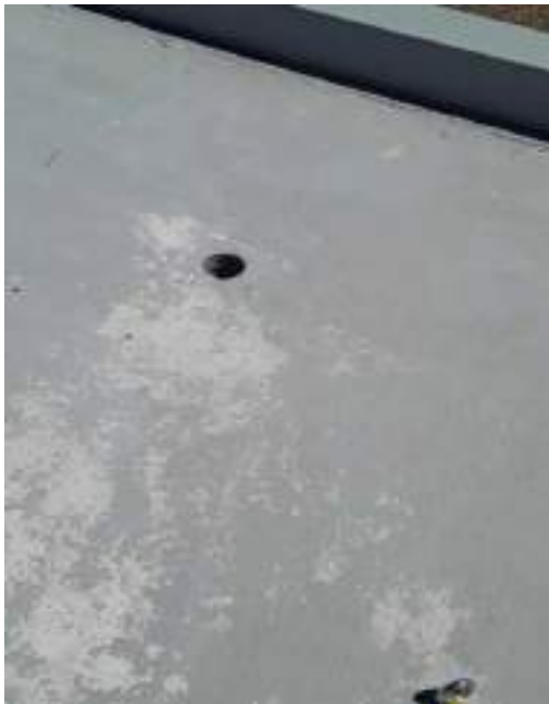
C 149- Building L roof, floor waste
