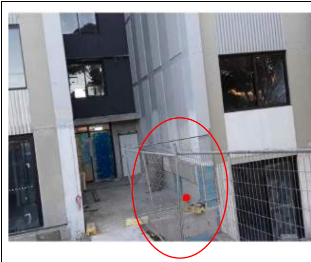
C 47 – South facade (Mitchell Avenue), Hebel cladding
