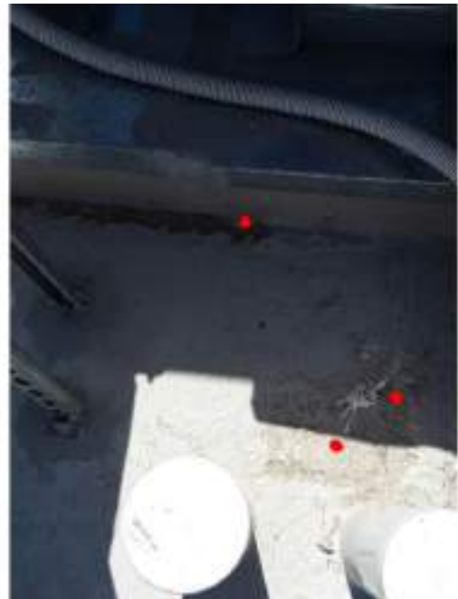
C 164 - Building U roof, concrete hob
