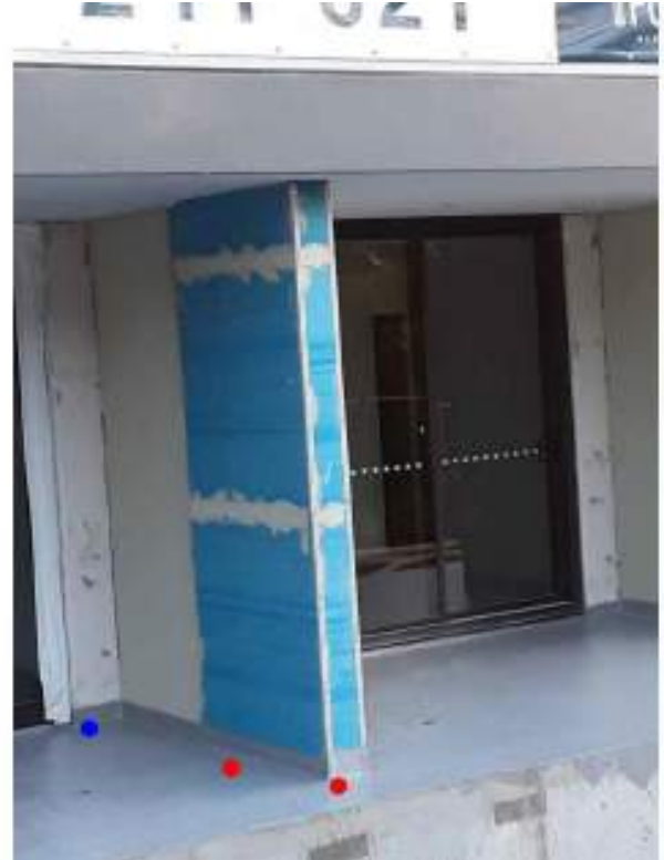
C 10 – East facade, unit balcony
