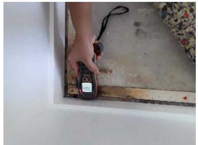
U G05.20 bedroom 2, wall (south-east corner)
