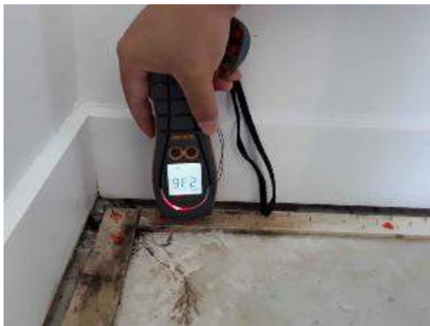
U G05.20 bedroom 2, wall (south-east corner)
