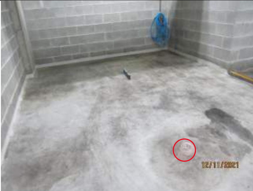
Zero fall indicated to eastern side of drainage inlet
