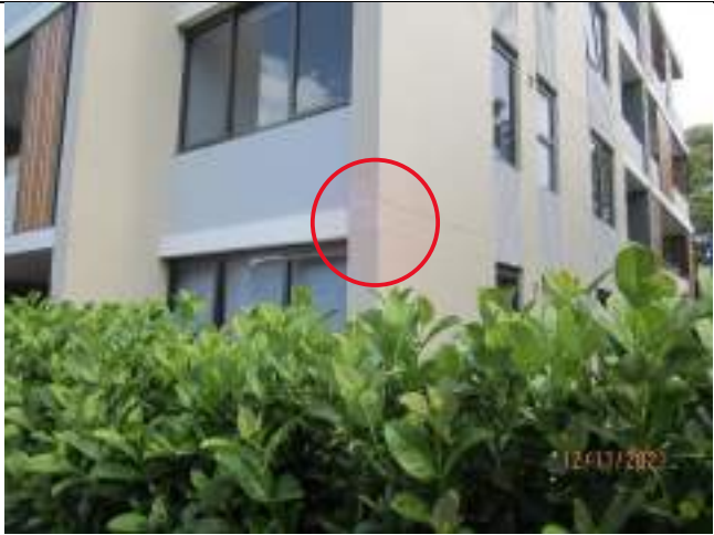
Evidence of moisture damage and repair carried out by Builder to column on northwestern corner of unit 106
