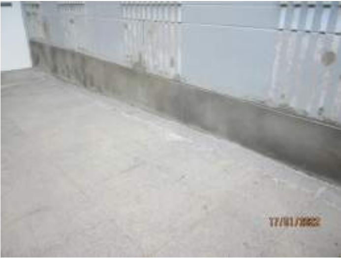
Render finish applied to waterproofing
