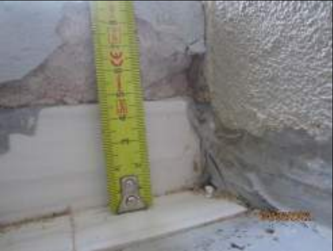
45mm PVC angle used at form upturn to waterproofing
