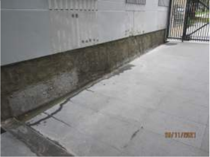
Render base coat applied to waterproofing membrane
