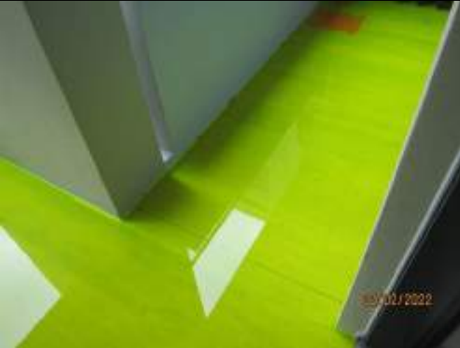
Flood testing using effluorescent dye to U107 Balcony
