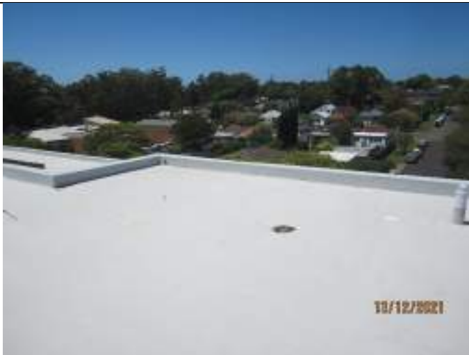
Southern side of roof Building U
