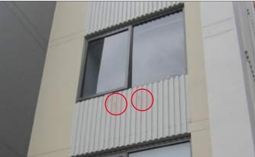
Evidence of corrosion to aerated concrete battening to upper levels on western side of main entry
