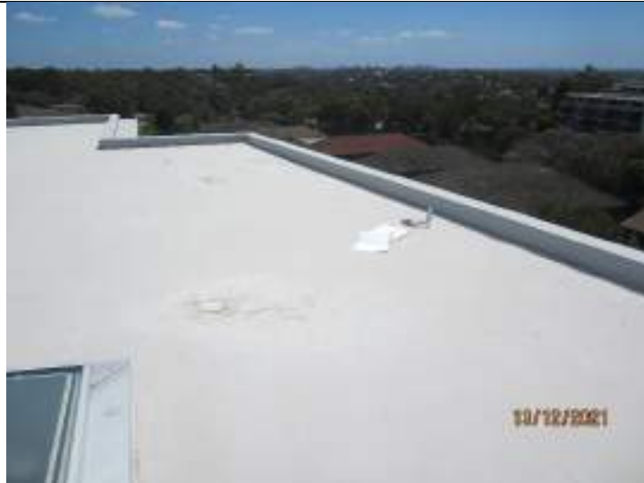
Building L south east side of roof
