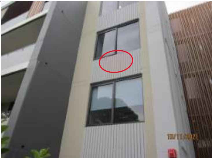
Location of corrosive fixings to aerated concrete battening on upper levels on western side of main entry
