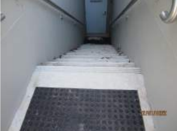
Drain located at base of external stairs Fire stair door
