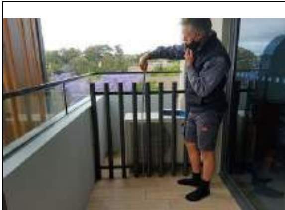
Unit 302 Air condition located on northeast corner of balcon
