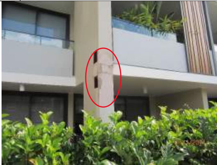
Evidence of destructive investigation carried out by Builder and moisture damage to eastern coloumn to unit G07 and unit 107
