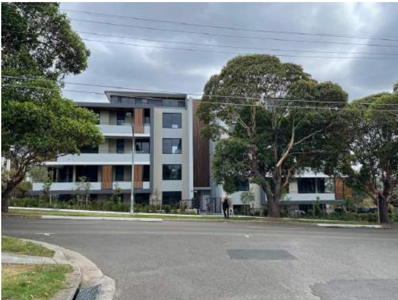
Photograph of front of building on Mitchell Street Jannali
