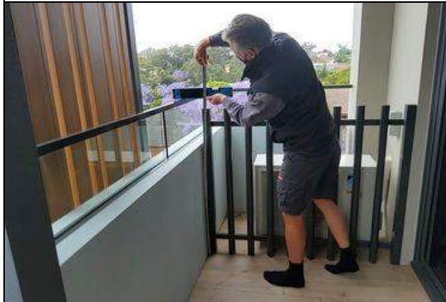
Unit 302 Height of balcony balustrade approximately 1140mm
