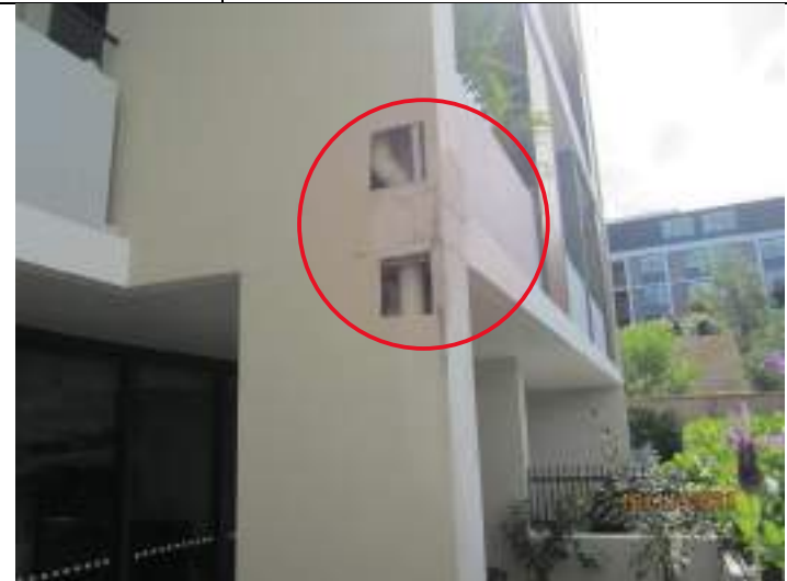
Evidence of destructive investigation carried out by Builder and moisture damage to eastern coloumn to unit G07 and unit 107
