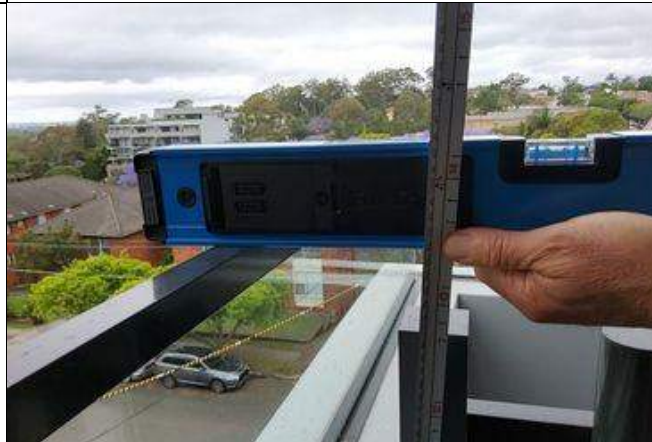
Unit 302 Height of balcony balustrade approximately 1140mm
