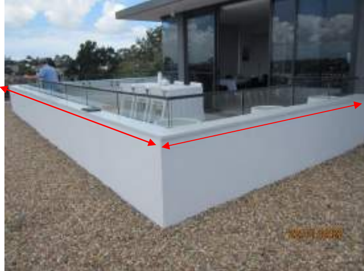
Image showing metal flashing installed to rendered balustrade to unit 401
