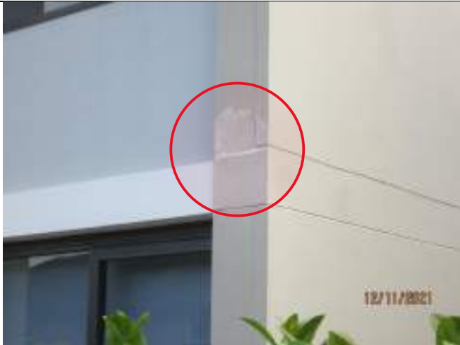
Evidence of moisture damage and repair carried out by Builder to column on northwestern corner of unit 106
