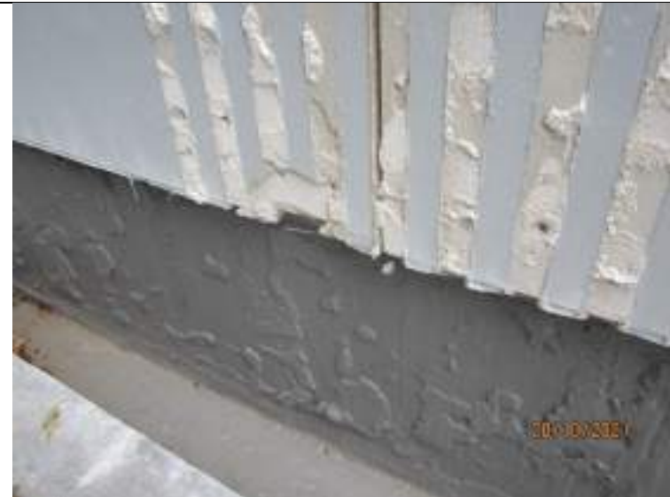
Waterproofing membrane applied over rough substrate
