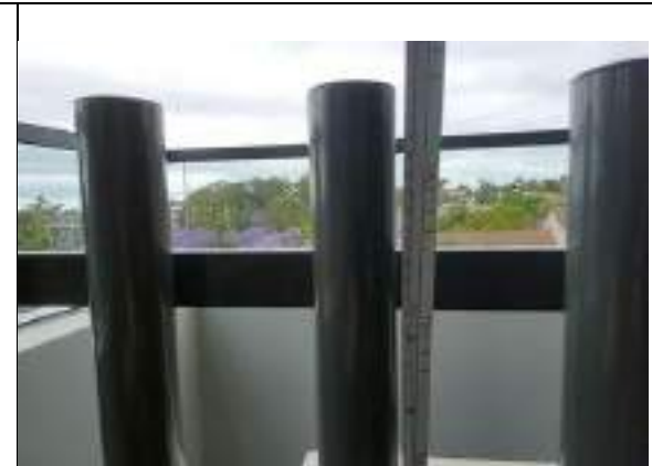
Unit 302 Height of top horizontal rail approximately 980mm
