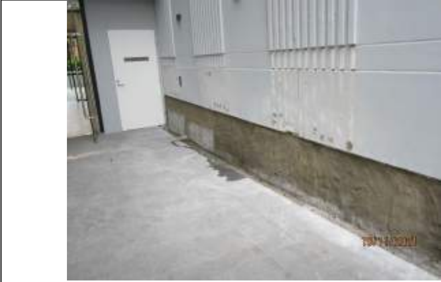
Render base coat applied to waterproofing membrane
