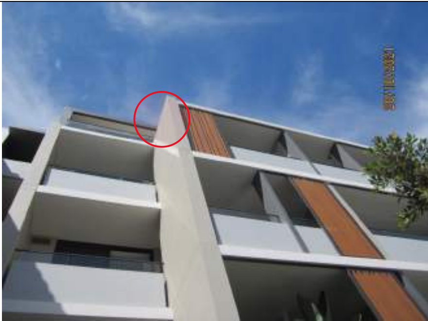
No flashing provided to top of columns on northern side of building. Evidence of efflorescence staining to eastern side of parapet.
