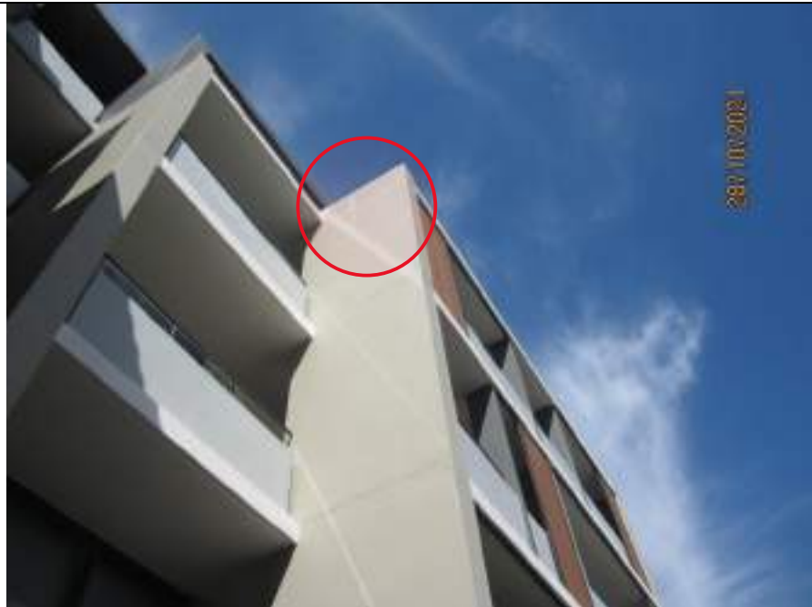
No flashing provided to top of columns on northern side of building. Evidence of efflorescence staining to eastern side of parapet.
