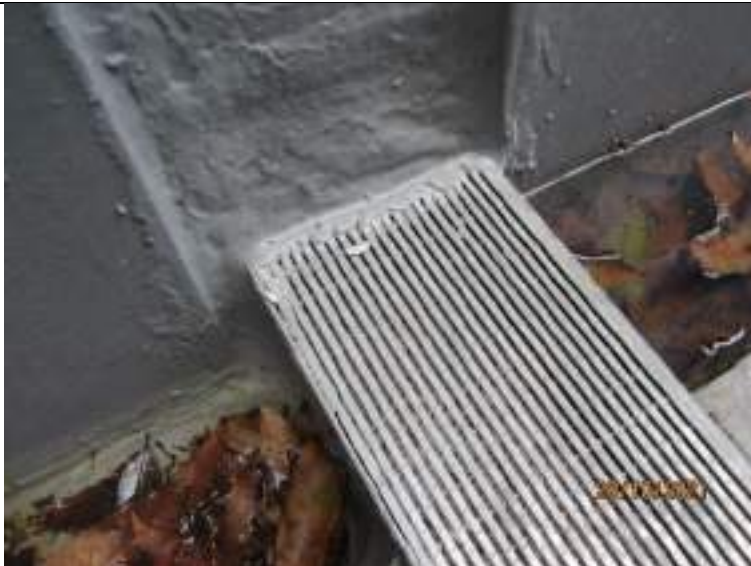
Waterproofing applied over stormwater grate
