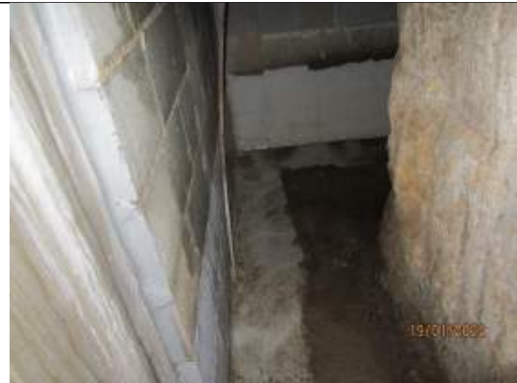
Waterproofing membrane terminated approximately 400mm above rear of southwestern wall
